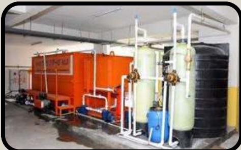
Sewage Treatment Plant
